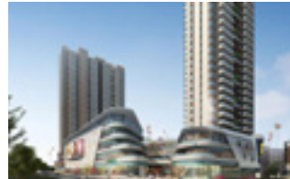
Chenzhou, Hunan Centro comercial Guiyang Plaza No. 1
